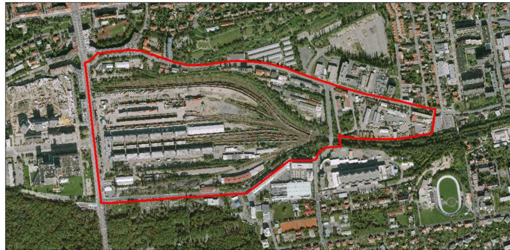
Figure 13 Overview of the Zizkov station location (ARNIKA, 2017)
