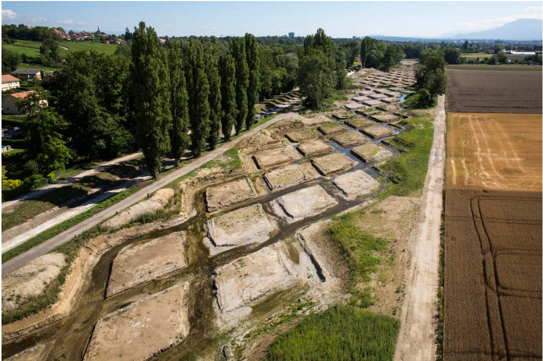
Figure 36. Renaturation of the river Aire Grid design contributes to variability in water regime and creates sandy aquatic environment which combines running and standing water regime biotope for many species. The self-restoration process support meanders and oxbow lakes formations scale, Restoring local aquatic biodiversity Source: Descombes and Rampini, 2016S http://www.landezine.com/wp-content/uploads/2016/06/09-Naturalization-river-channel-landscape-architecture-Fabio-Chironi-300x300.jpg
