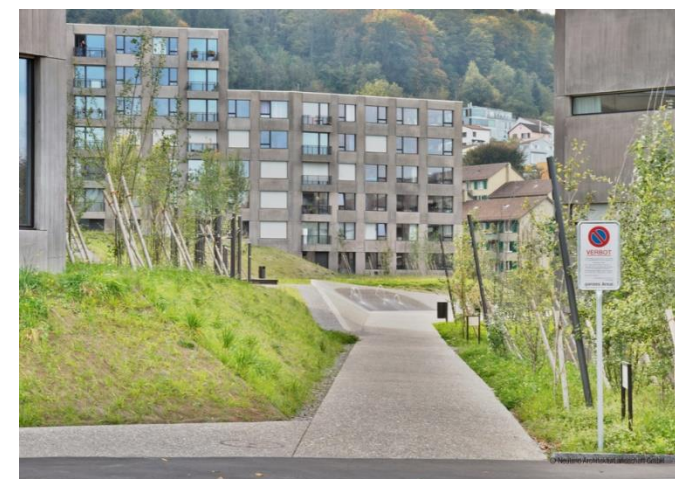
Obr. 17 - Pohled do vnitrobloku Trimeli (zdroj: http://www.landezine.com/index.php/2015/05/housing-project-triemli/ )
