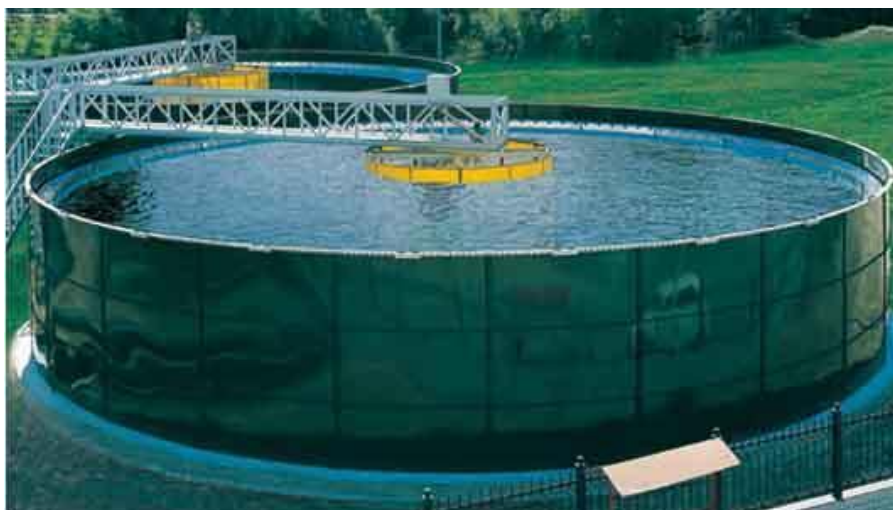
Obr. 16: Závlahová nádrž, Zdroj: http://www.cectanks.com/sale-7587549-agricultural-water-storage-tanks-for-irrigation-enamel-100-000-gallon-gfts-tank.html
