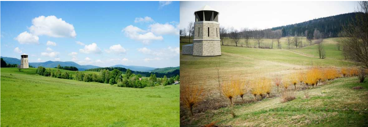
Fig. 4. Wind turbine presenting the structure of historic view tower, located in “Jizerské hory” region and in “Krkonoše” region, Northern Bohemia, Czech Republic.
