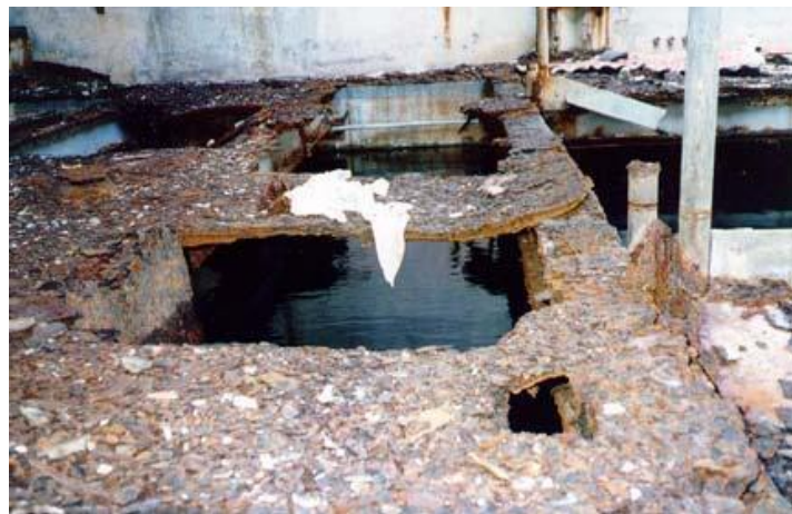
Figure 1.10: Uniform corrosion occurs without protective coating. [5]
