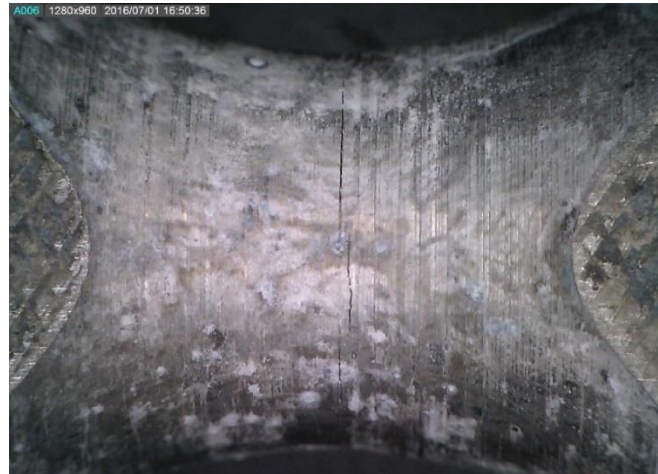
Figure 4.39: Initial cracks found on surface of specimen at notched area.
