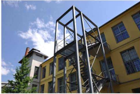
The Emergency staircase
