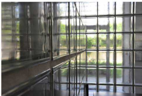
The Wall of glazed bricks
