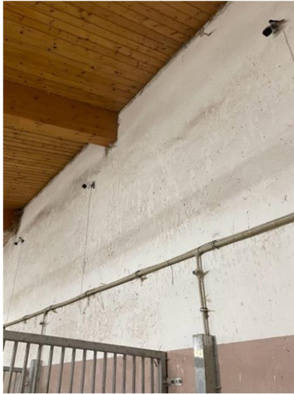
Figure 1: Placement of cameras on the wall
