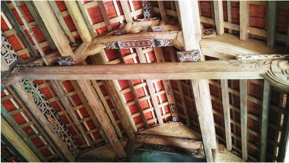
Figure IV. Ornamental roof construction made from X. noronhianum
