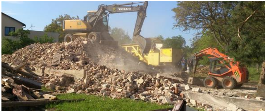
Figure 24: Company in Plzeň specializing in demolition and following sorting and crushing
