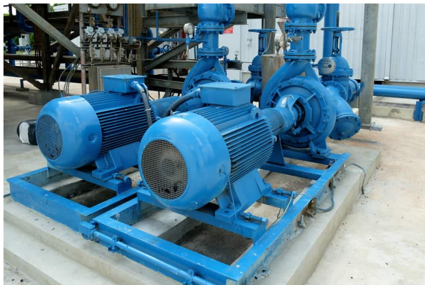
Figure 6 Centrifugal Pump (Lauren Cella, 2020)
