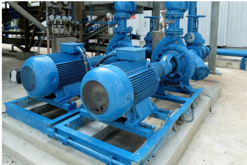
Figure 6 Centrifugal Pump (Lauren Cella, 2020)
