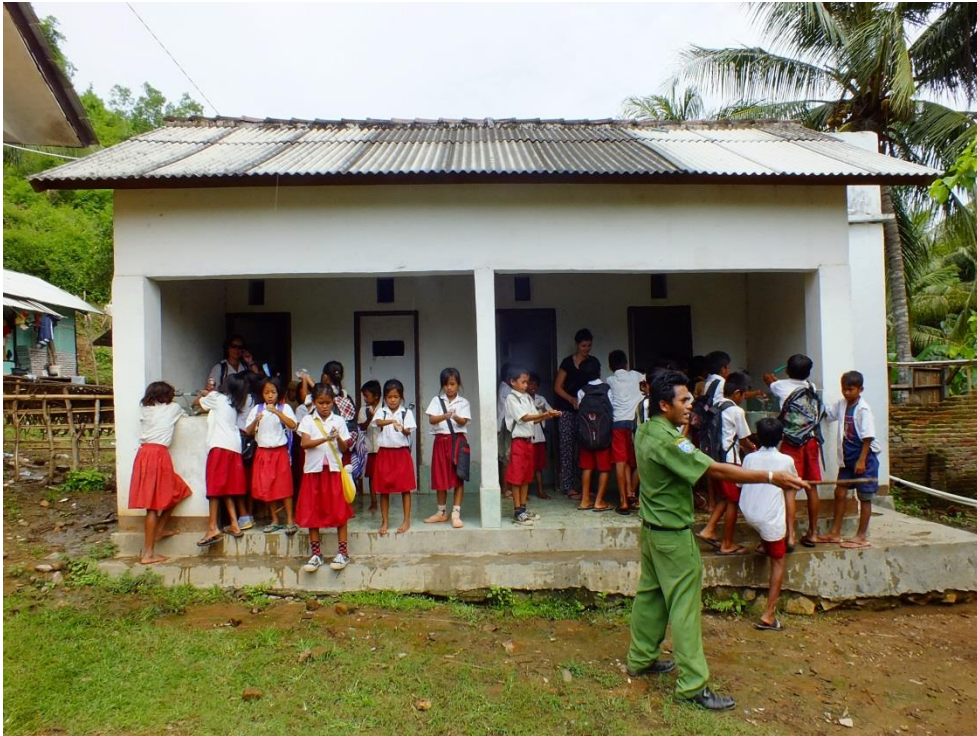
Annex 5: Sanitary facilities built within a DP Kintari organization. Ngolang, Lombok
