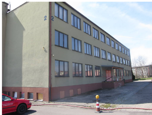
Figure D.2: The building from the experiment (north-east view).
