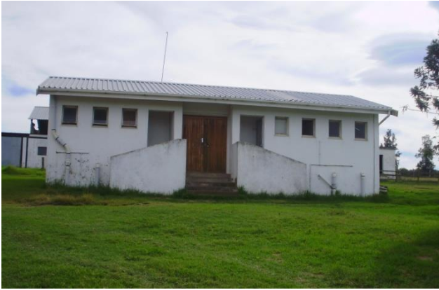
Figure 14: Building suitable for teaching of theory, Source: author's archive
