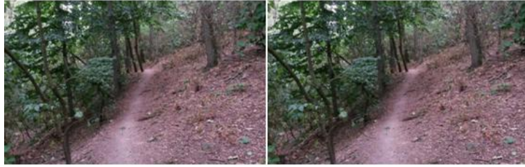
Figure 24 - Example of trail that follows contour at Wild Sarka Study area. This facilitates trail drainage and at the same time confines users to trail without diverging to the vegetation. (Photographs by Phaniel Gade)
