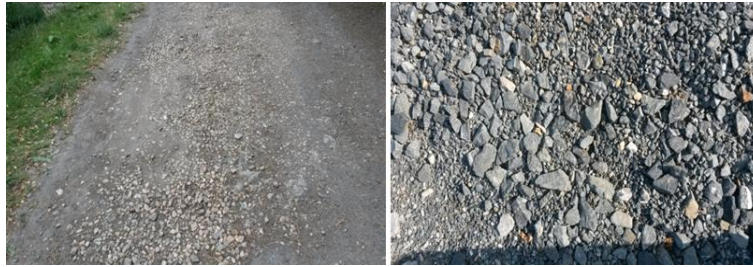
Figure 26 - Example of crushed gravels that can be used minimizes the rate of erosion in degraded segments of trails. (Photographs by Phaniel Gade)
