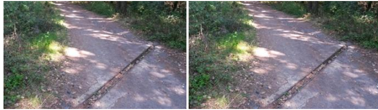
Figure 19- Example of constructed water bar on trail segments in Ďáblický háj and Wild Šárka urban forest, which can reduce erosion on trail by routing run off away from trail
