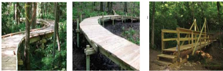
Figure 25 - Examples of constructed boardwalks which can facilitate protection of urban forest understory vegetation and also provide easy access through standing waters or muddy spots (Manual and guide for trail design)
