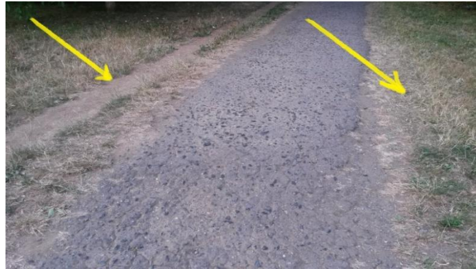
Figure 14 An urban forest paved trail without constructed trail side-hill, which result to outer-boundary disturbances as users venture off the trails. (Photographs by Phaniel Gade)
