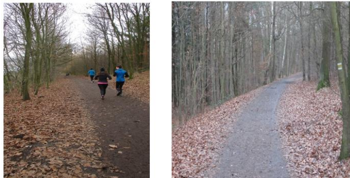
Figure 15 - Example of trail with flatter side-slope at Ďáblický forest which offers low resistant trail widening as well as little resistant to prevent or obstruct the drainage of water from incised trail treads. This can also encourage proliferation of unauthorized trails because of open meadows at trail side.
