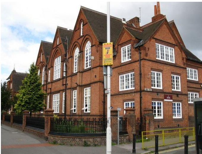
(School Building, Oxford Road, 2009)
