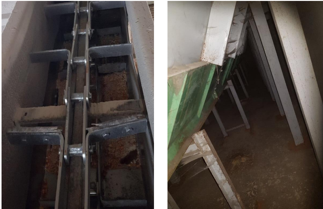
Fig. 5.2: Chain Conveyor measuring points (Photo by author, 2023)
