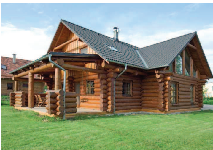
Obr. 2.8 – Srubová stavba [15]
