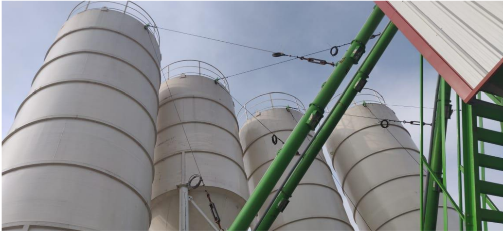
Figure 4: Cement Silo in The Organisation [20]
