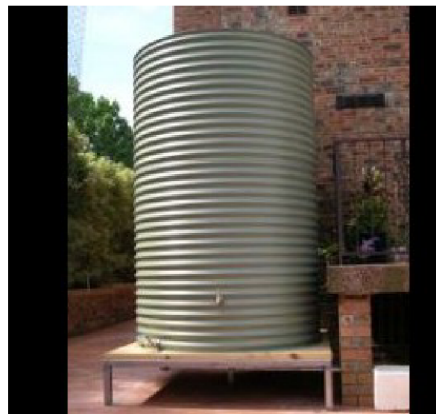
Fig. 10 Steel water storage tank (43)
