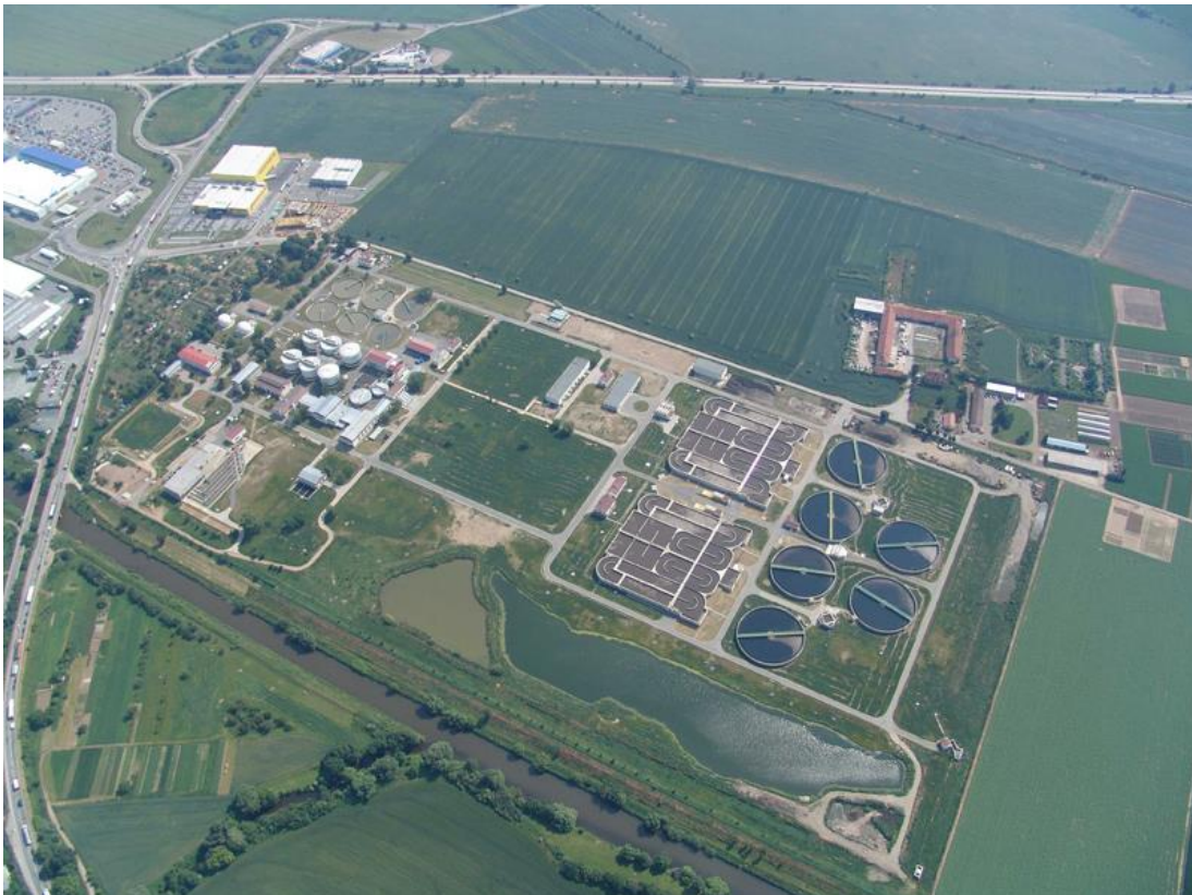
Figure 59: General view to the area WWTP Modřice. [60]
