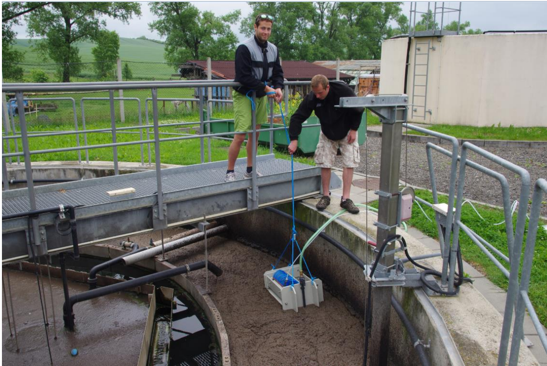
Figure 47: launching MBR module into the tank with activated sludge, WWTP Letonice
