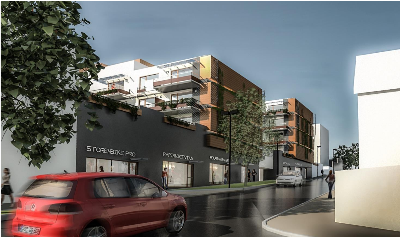
Figure 33: Street view picture of Nádražní 23 project
