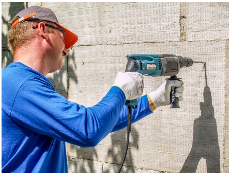
Obr. 12 Vŕtanie diery pre kotvu [2]
