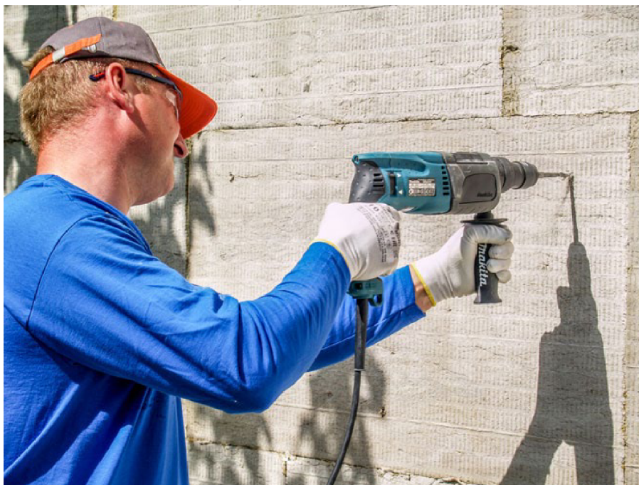
Obr. 12 Vrtanie diery pre kotvu [2]
