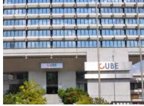
CUBE OFFICE CENTER
