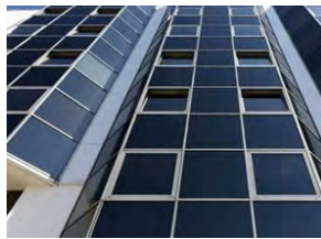
AIRPORT BUSINESS CENTRE
