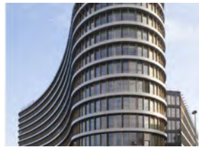
ENTERPRISE OFFICE CENTER
