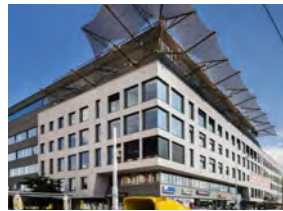
FACTORY OFFICE CENTRE
