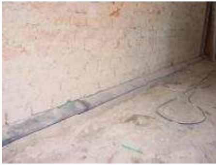
Obr. 7.1.7: hydroizolace
