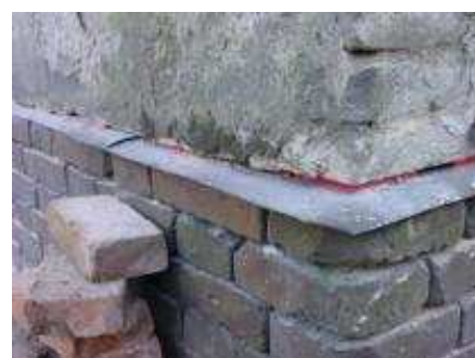
Obr. 7.1.6: hydroizolace
