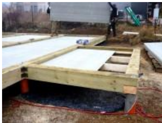
Obr 22 Crawl Space (PB24, 2016)
