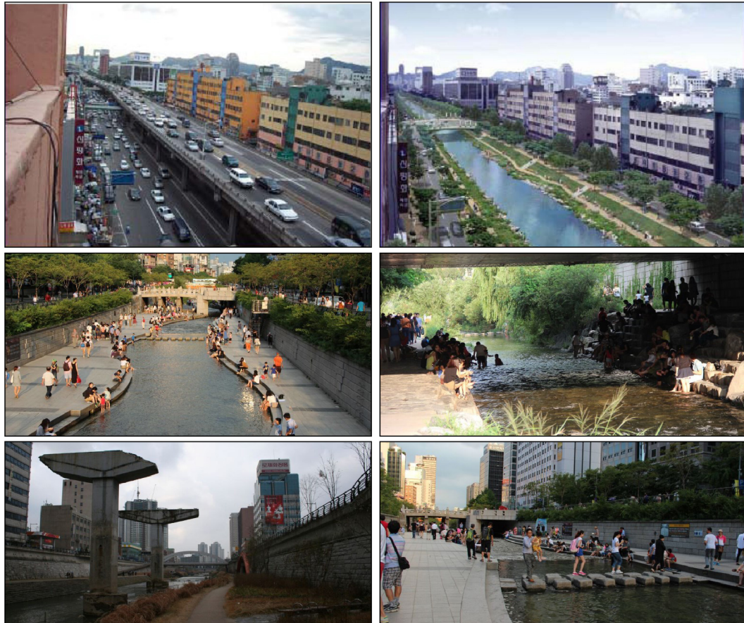
Figure 4.8: Cheonggyecheon, before and after of GBI implementation ( Research center director of Seoul development institute, 2002 ).
