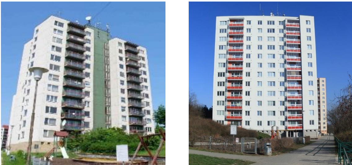
Figure 26. Koniklecová 4 block of flats: Eastern view (left) shows state of the building before the 2010 renovation, Western view (right) shows state of the building after renovation. (Mørck, 2017)
