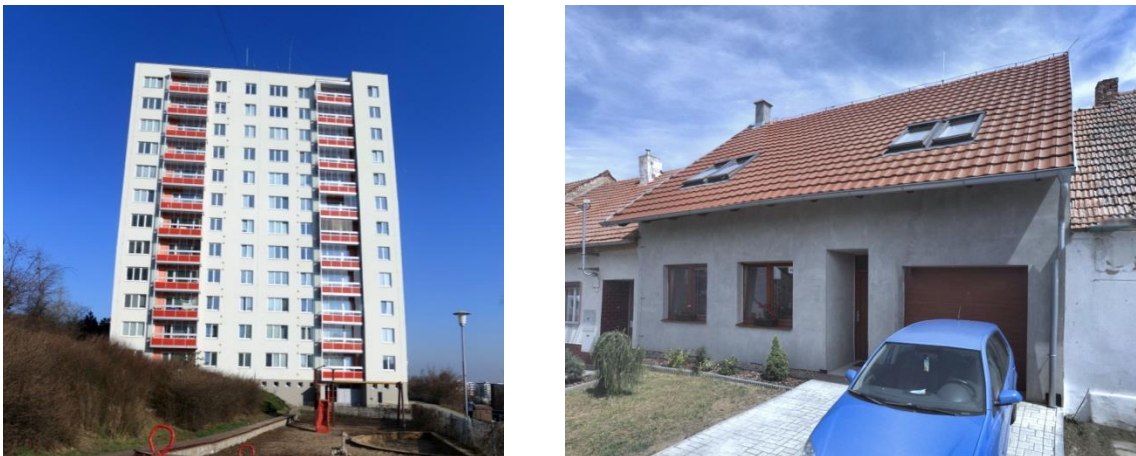
Figure 21. Photographs of both case studies after renovation (construction). Koniklecová 4 block-of-flats is on the left, Přebice 442 single-family house is on the right, (Mapy.cz, 2017).
