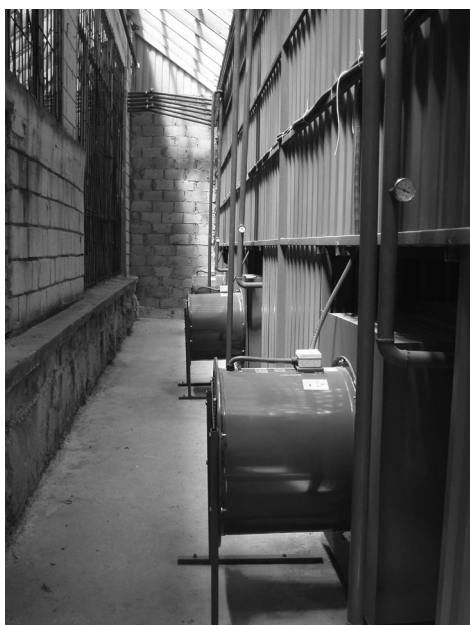
Fig. 3. Mixing chamber with reversible fans
