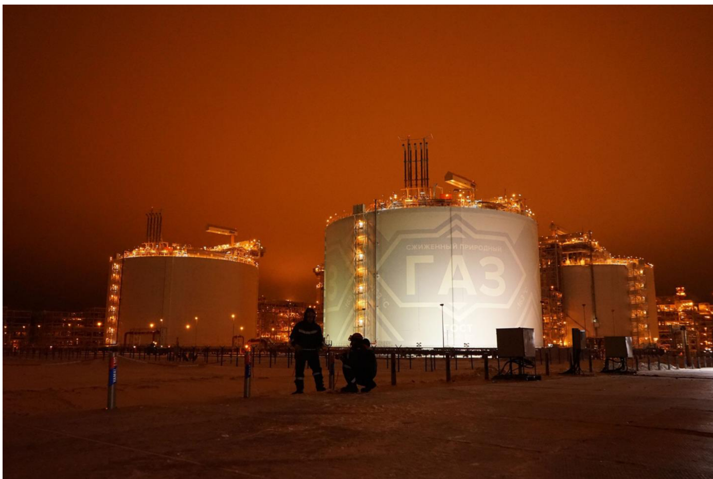
South Tanbey LNG – the biggest LNG plant up the Arctic circle / Polar Night. The red color of the sky is because of HP Flare (750 – 800 Celsius)
