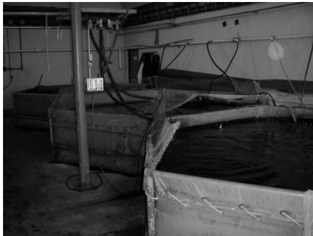
Fig. 10. Rearing hall of the farm in Mydlovary (currently, rented by BaHa, Ltd company). Photo by J. Kouřil
