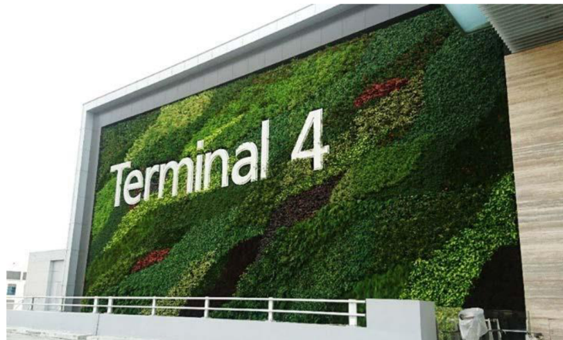
Figure 5 Modular Green Wall at Changi Airport, Singapore (GWSLivingArt.com)
