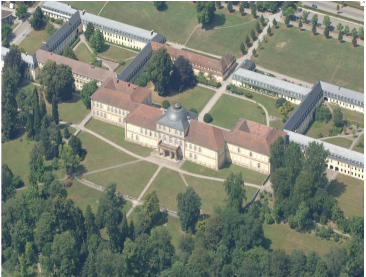
Aerial photo of Hohenheim Castle Park or Garden(uni-hohenheim.de)
