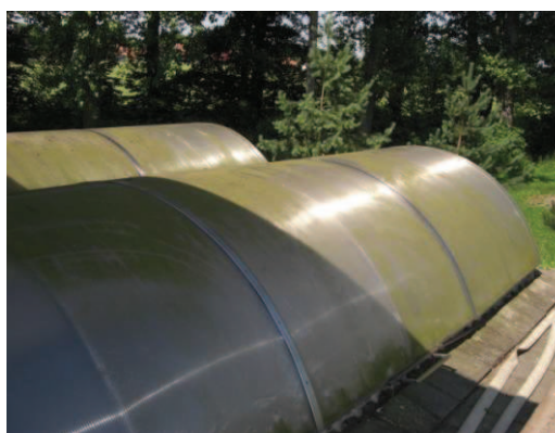
Obr. 34 SBR reaktory
