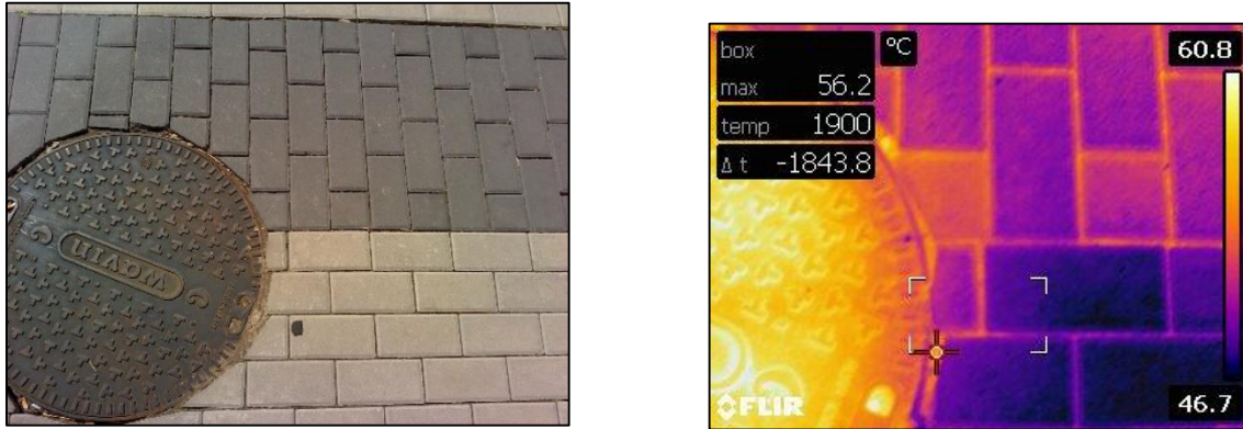
Figure 55. Visible and infrared image of dark and light tile, with Iron Drainage Covers (19 June 2022, at 14.06).
