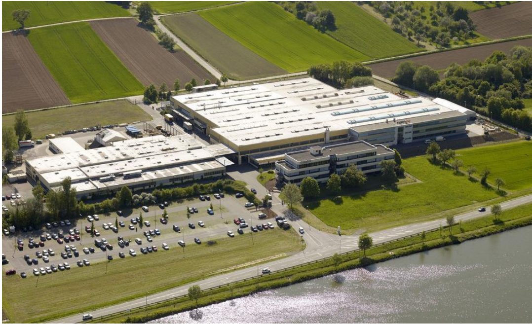
Figure 1 - FLT Headquarters in Haßmersheim [11]
