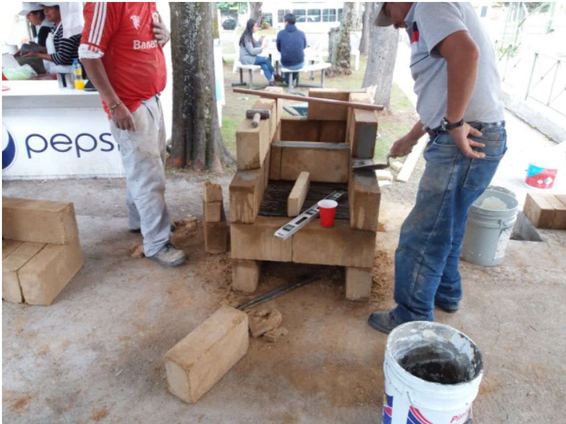
Fig 2-4 Building of the stove with a detail on bricks and adhesive
