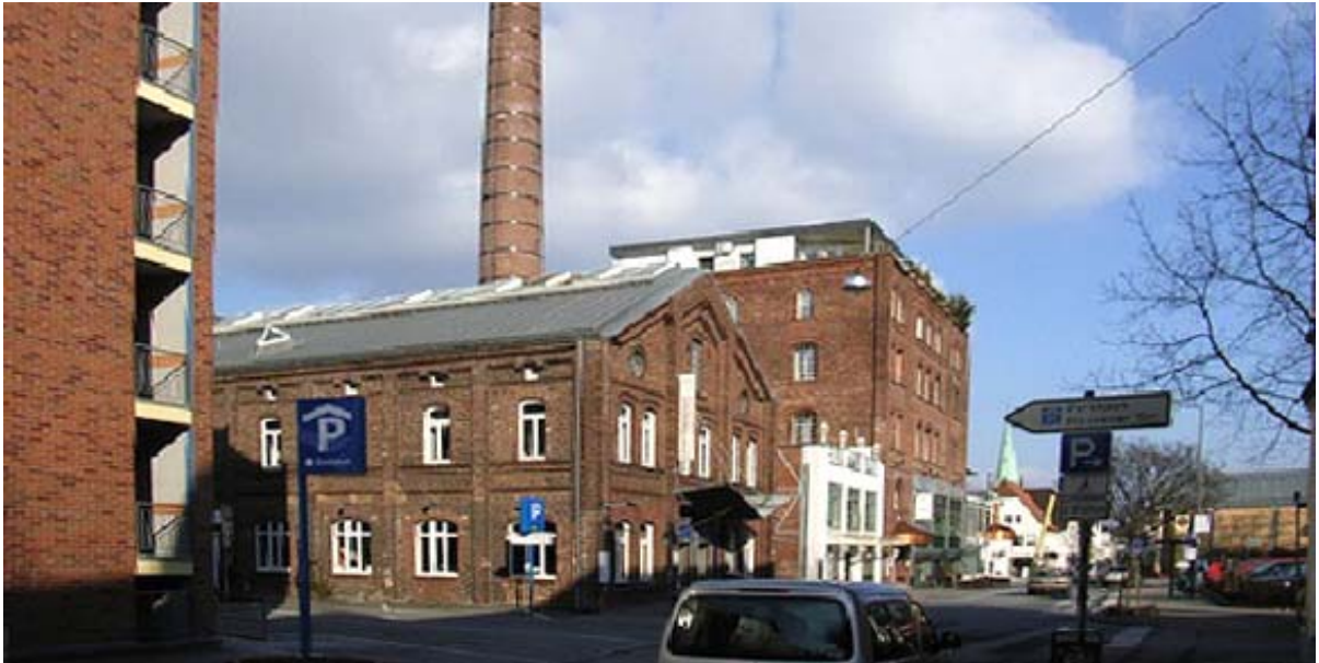
Obr. 44: Pohled na Centre for International Light Art, Unna, 2002 113
