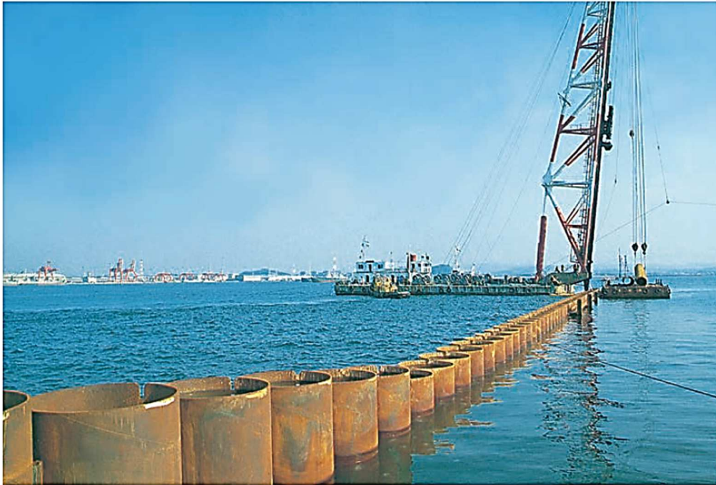
Figure 1.2 Construction of Interlocking Pipe Pile Wall [2]
