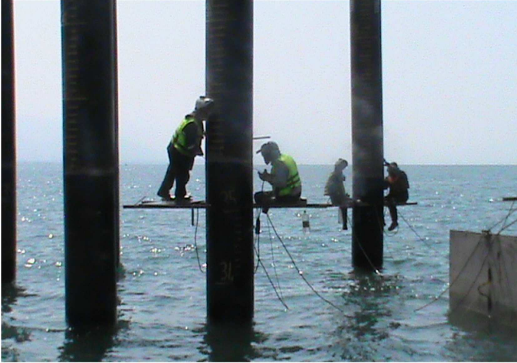
Figure 1.4 Pile Works on the Sea [3]
