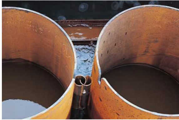
Figure 1.3 Detail of the interlock [2]
