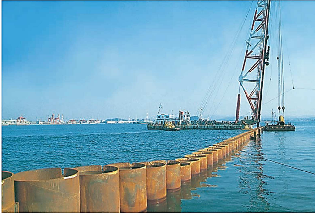
Figure 1.2 Construction of Interlocking Pipe Pile Wall [2]
