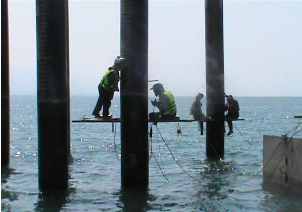
Figure 1.4 Pile Works on the Sea [3]
