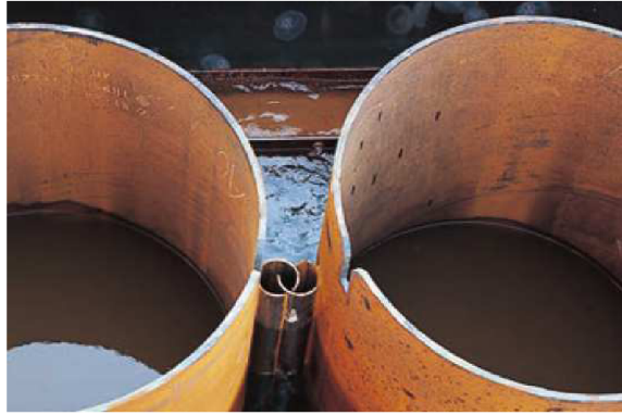
Figure 1.3 Detail of the interlock [2]
