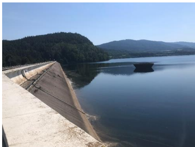
Figure 7. The dam and the overflow shaft of the water reservoir Nýrsko (author's archive)
