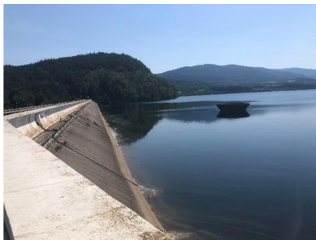
Figure 7. The dam and the overflow shaft of the water reservoir Nýrsko (author's archive)
