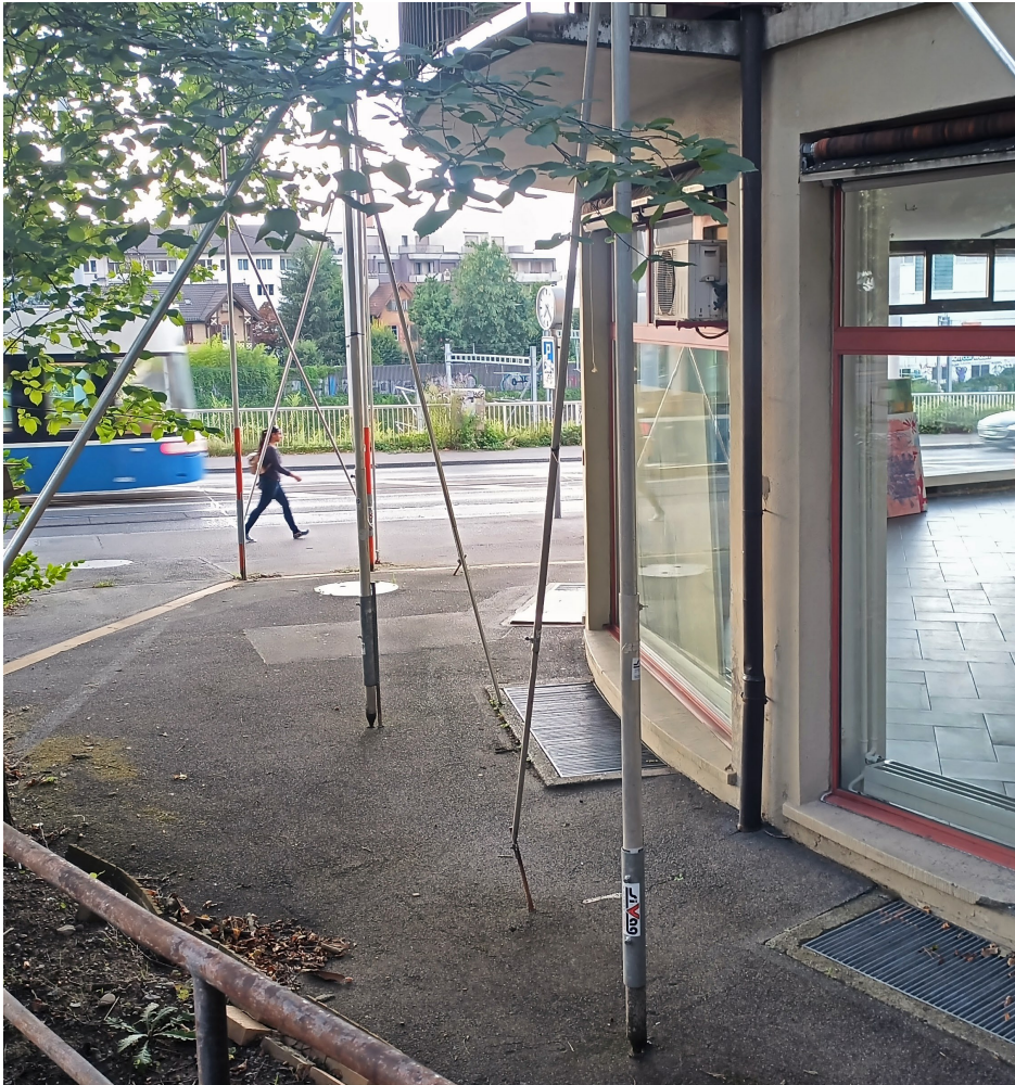
Figure 9: Photo depicting how citizens of Zurich are informed through Baugespann of future development projects in situ
