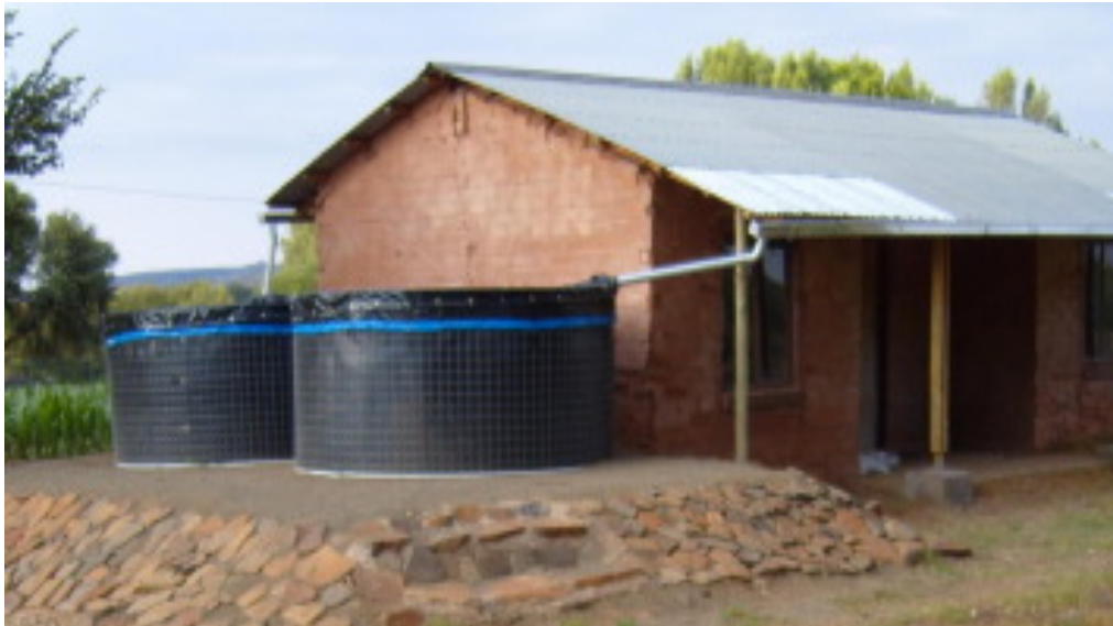
Figure 4 domestic RWH aboveground (Mwenge Kahinda & Taigbenu 2011)
