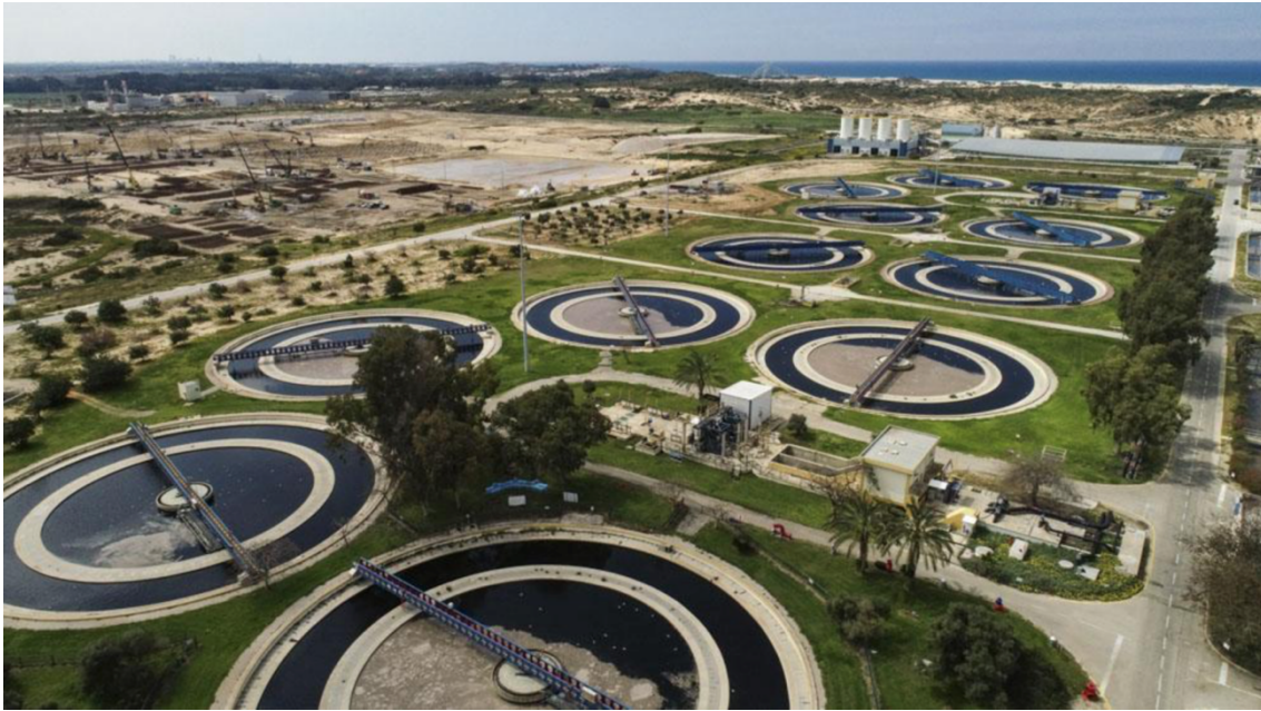
Figure 19 Shafdan wastewater treatment plant (“The Shafdan R&D Center – An open installation for wastewater treatment and effluent reclamation solutions - Global Water Intelligence” 2020)
