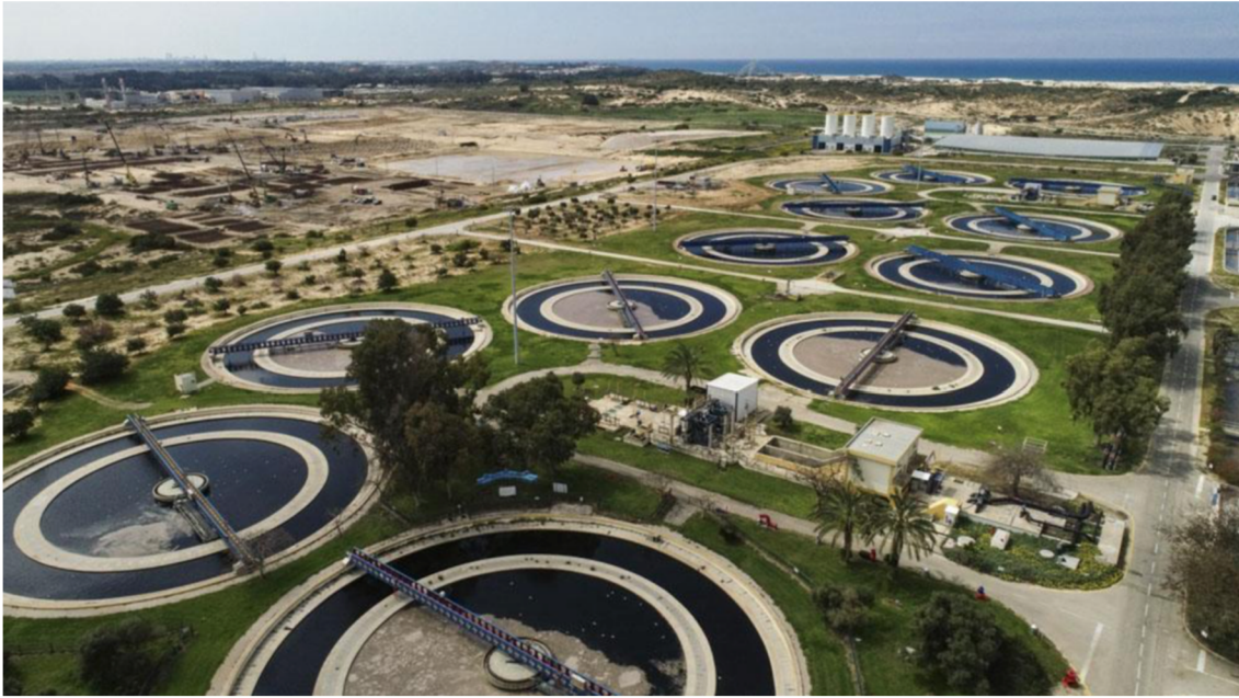
Figure 19 Shafdan wastewater treatment plant (“The Shafdan R&D Center – An open installation for wastewater treatment and effluent reclamation solutions - Global Water Intelligence” 2020)
