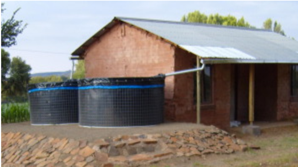
Figure 4 domestic RWH aboveground (Mwenge Kahinda & Taigbenu 2011)
