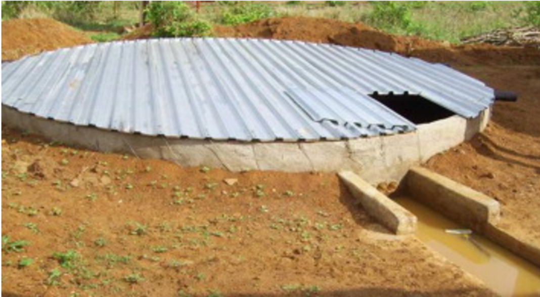
Figure 5 domestic RWH underground (Mwenge Kahinda & Taigbenu 2011)
