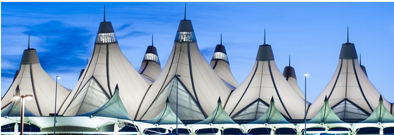
Fig. 2 Roof of Denver International Airport, USA [III]
