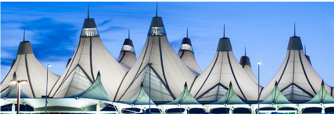
Fig. 2 Roof of Denver International Airport, USA [III]
