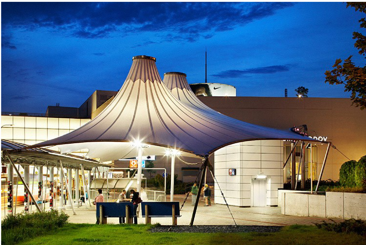
Fig. 29 Shopping Centre Chodov in Prague (East Exit from Metro), Czech Republic [VI]
