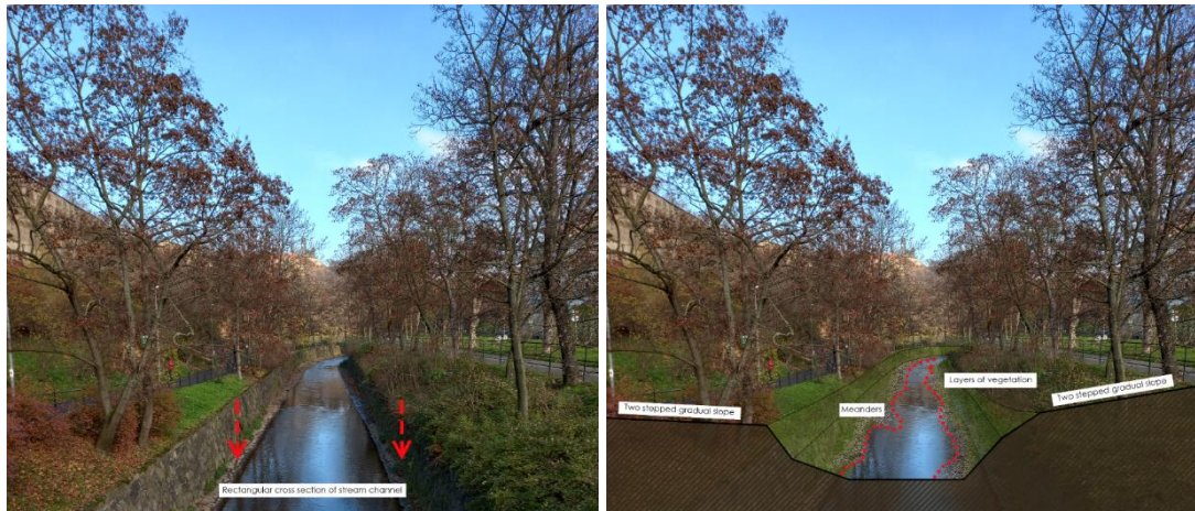
Figure 47. Example 2 – observation and proposed solution at creek channel in Folimanka Park area. Source: Author
