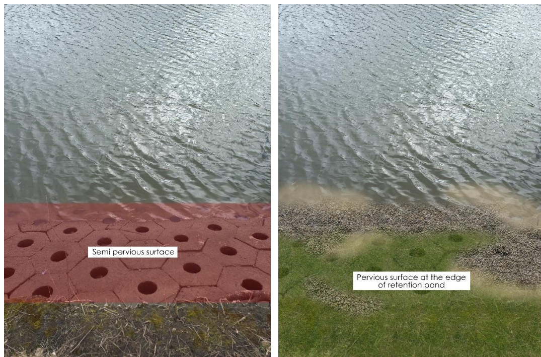
Figure 51. Example 2 – Observation of semi-pervious surface at the pond banks and Proposed solution of textural change, respectively, at Hamerský pond. Source: Author
